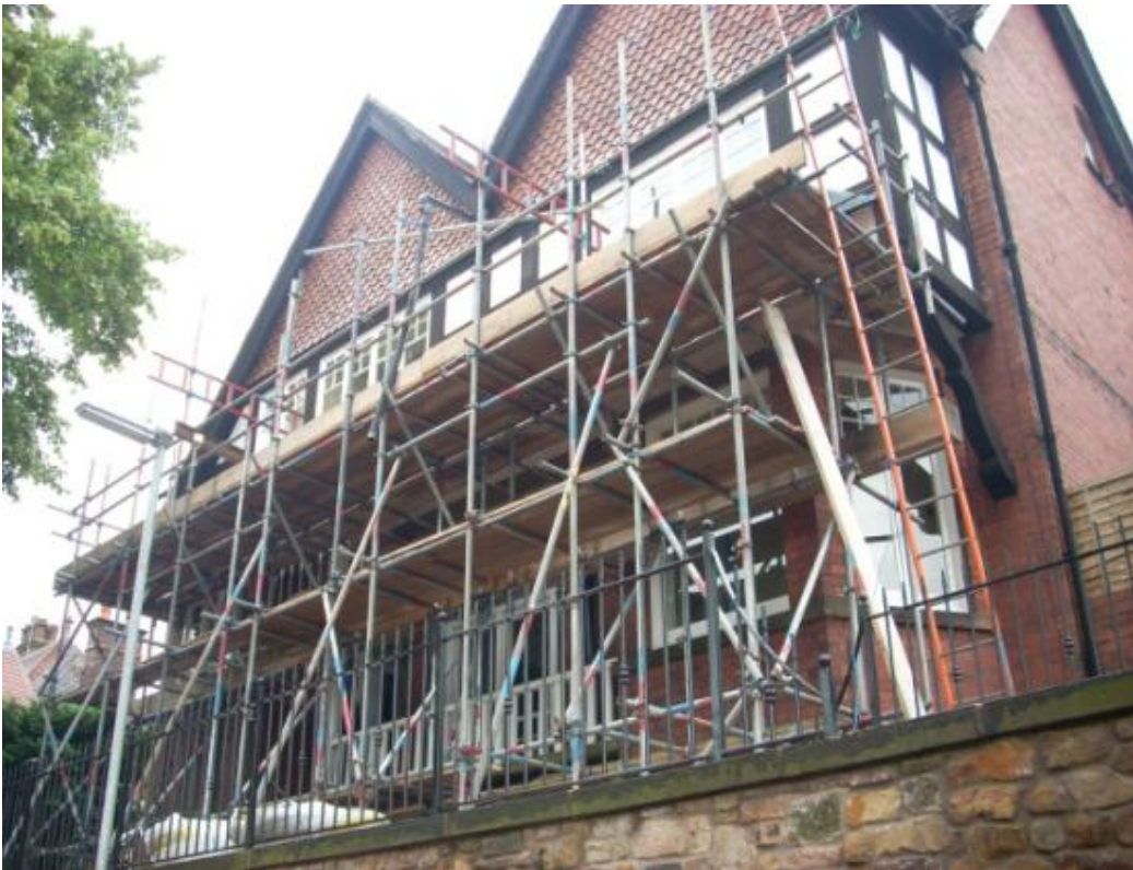
TEMPORARY SUPPORT SCAFFOLD – WORKS IN PROGRESS
