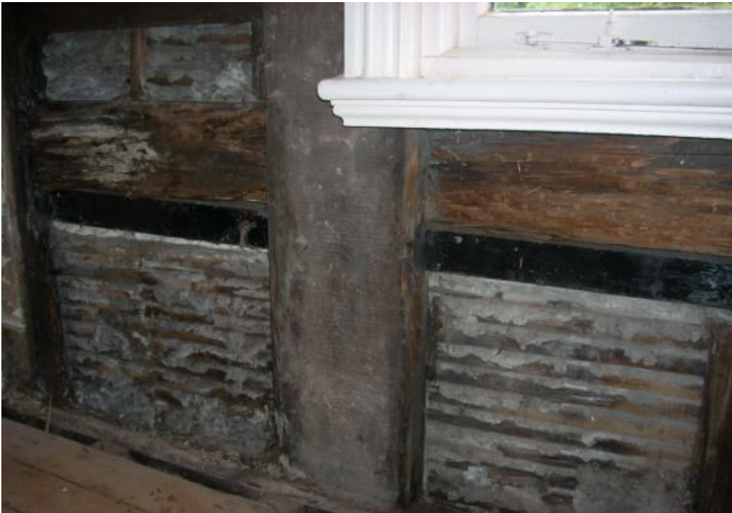
PART EXPOSURE OF UPPER TIMBER FRAME AND SOLE PLATE BEAM
