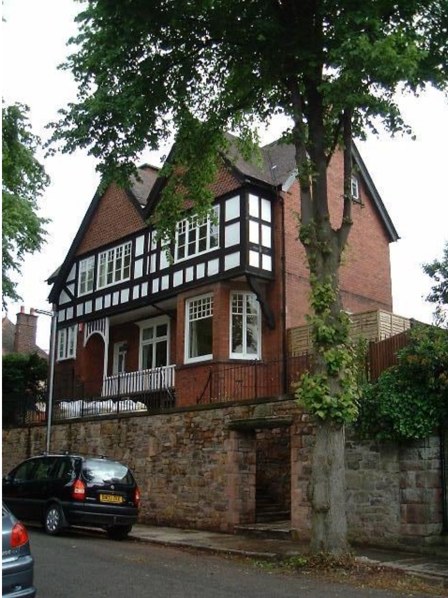
FRONT CORNER ELEVATION PRIOR TO WORKS
